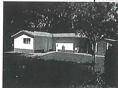
Kitchen, storage and meeting area
