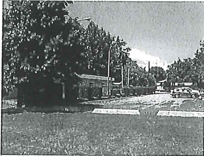
South east corner and view of the parking lot.
